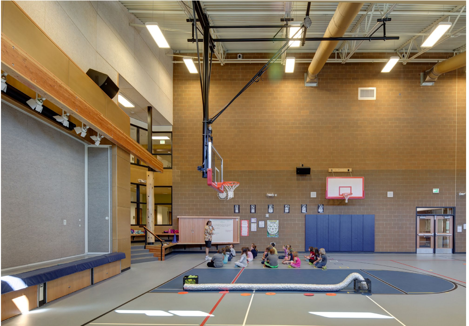
Structural masonry walls in the gym and other areas also afford the benefit of attractive, durable surfaces without adding finish material.
