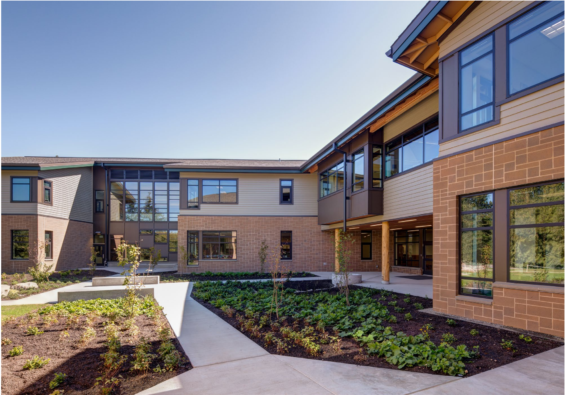
In the courtyard, varying sized masonry units create visual interest and give the walls a sense of scale.
